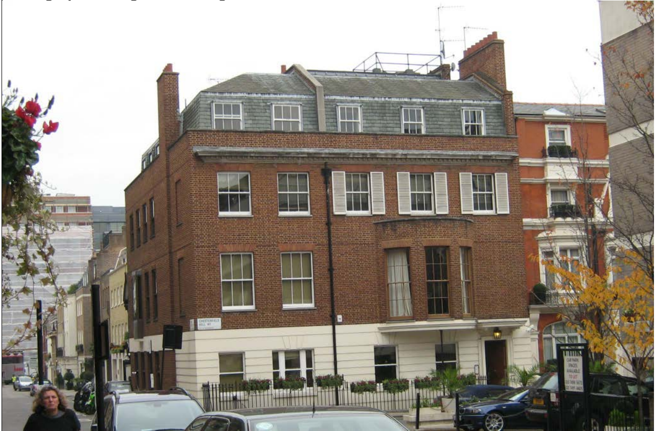
Photograph 1: Original building before demolition
